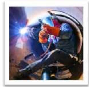
**Air replacement:** Provide adequate ventilation to all welding and cutting operations in confined spaces to prevent the accumulation of toxic materials or possible oxygen deficiency. The welder, helpers, and other personnel in the immediate vicinity must get adequate clean and respirable ventilation.
